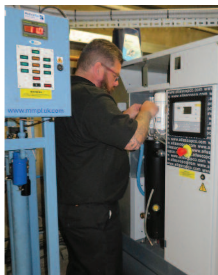
Adam Clark servicing a compressor.
