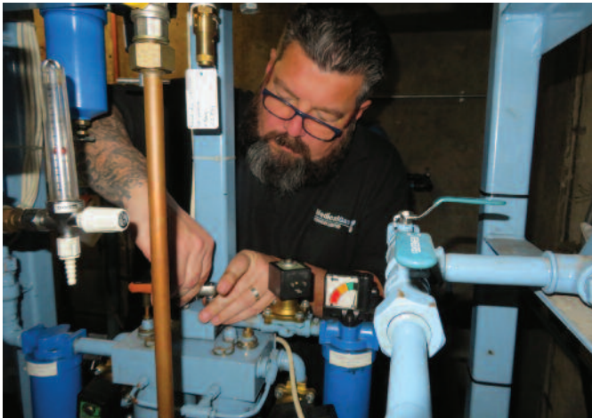
Adam Clark undertaking a dryer service.
