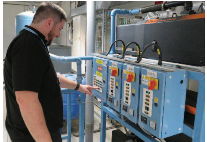
Ryan Clark carrying out the PPM on a vacuum plant.
