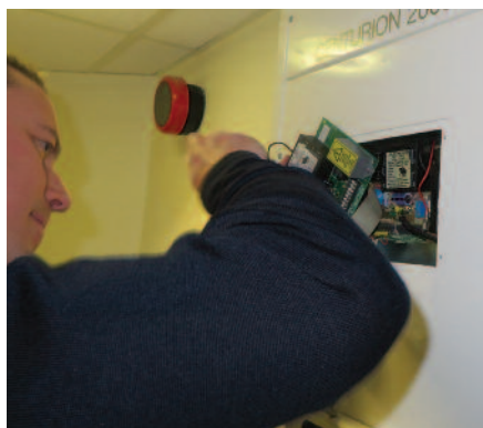
Stephen Hutchings repairing a local alarm panel.
