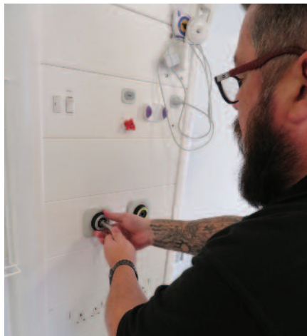
Adam Clark servicing a terminal unit.
