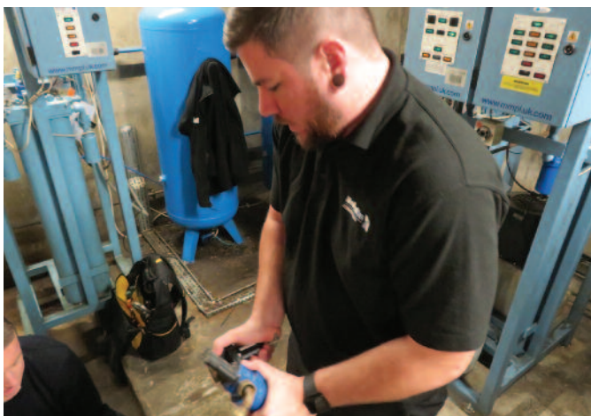
Ryan Clark repairing an air filter.
